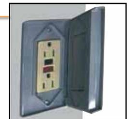
120V GFI duplex receptacle, located on the side of the panel, provides auxiliary power for other devices.
